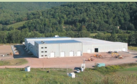
Delaware County Facility, NY (USA)
